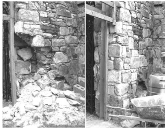
Left: Southeast corner before. Right: Stonework done.
