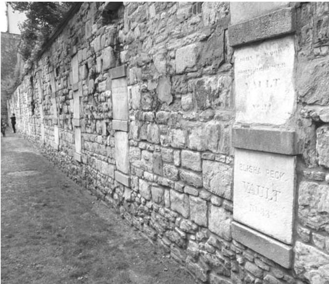
The South Wall of the Cemetery has been completely repointed this year from below ground level to about four feet above ground.
