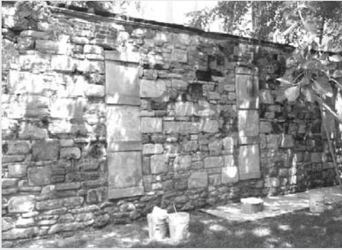
The existing eastern portion of the North Wall of the Cemetery with repointing work in progress.
